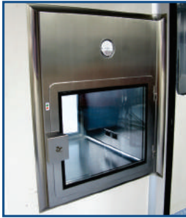
Pass Through Ventilado
